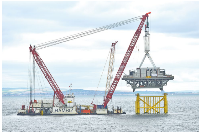
Installation of offshore substation platform
