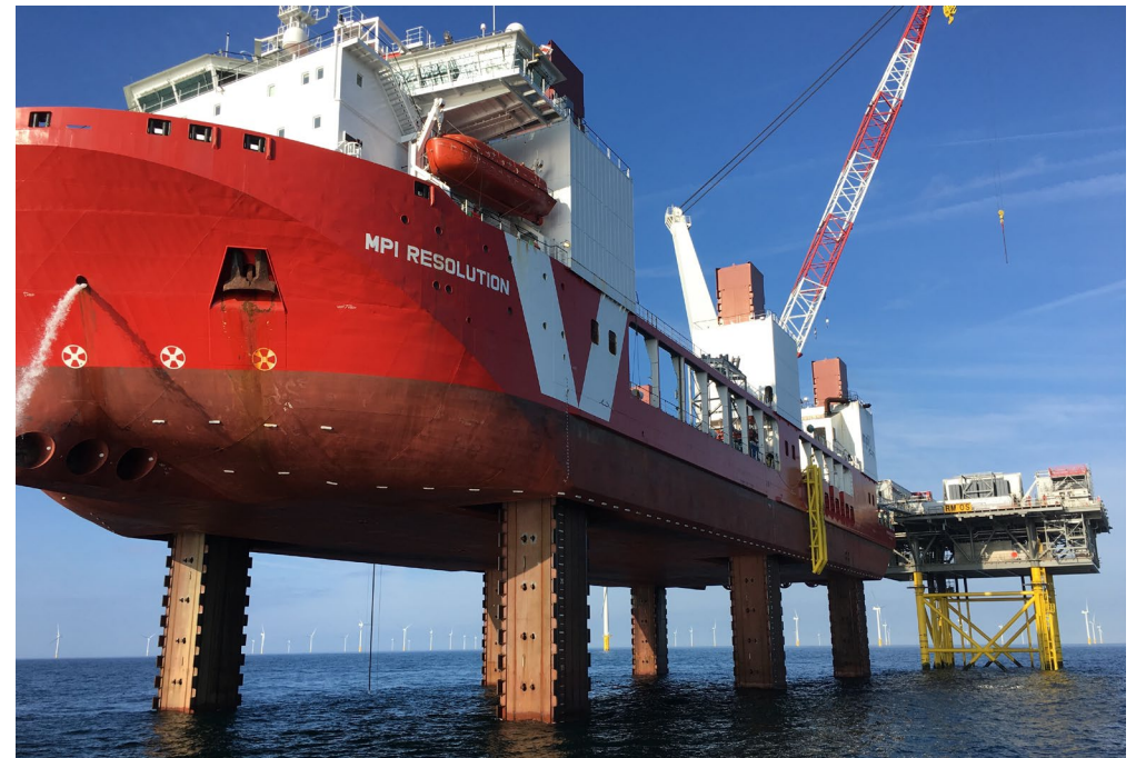
Commissioning of substation equipment
