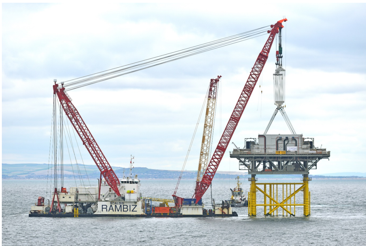
Graphic 4-10 Example offshore substation during installation (Rampion 1 offshore wind farm)
