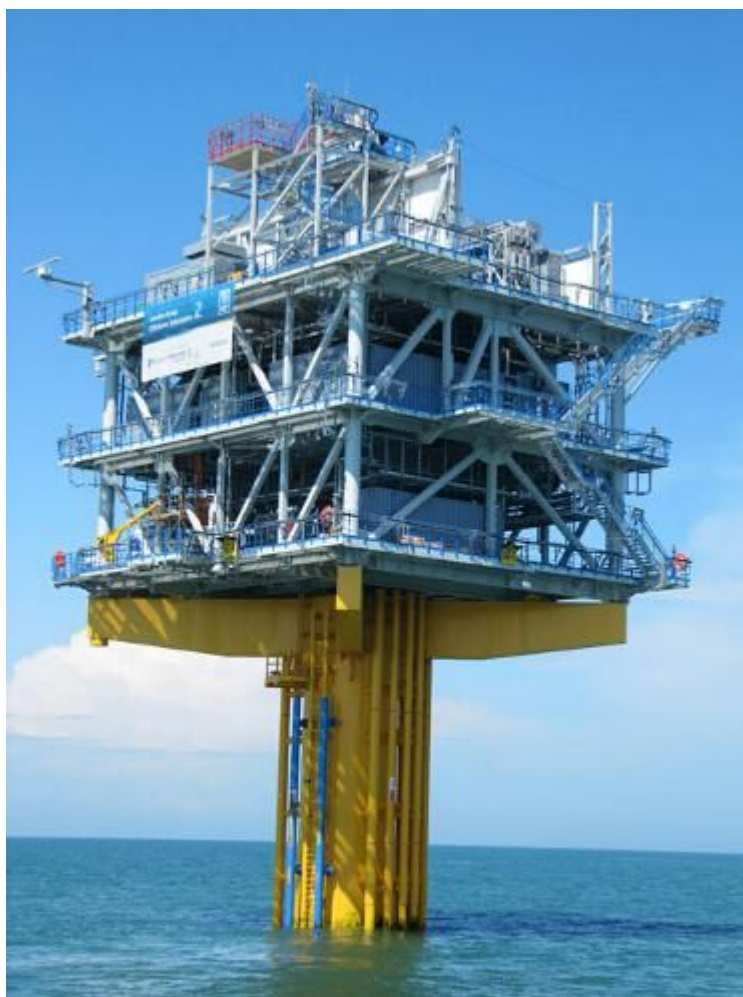
Graphic 4-8 Example offshore substation with monopile foundation (London Array offshore wind farm)
