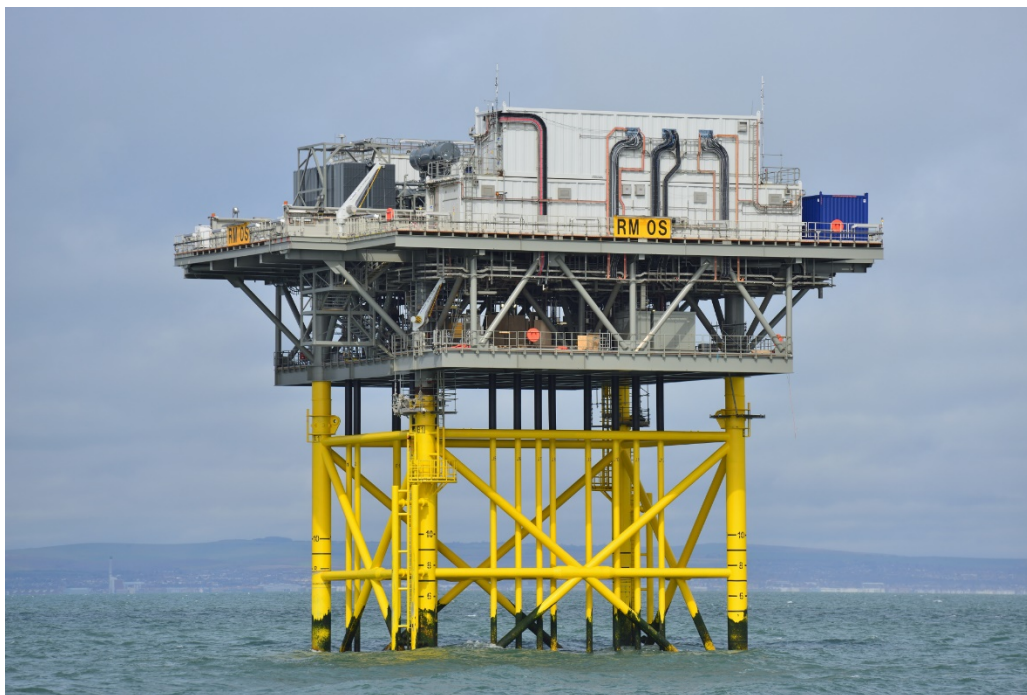
Graphic 4-9 Offshore substation with four-legged jacket piled foundation example
