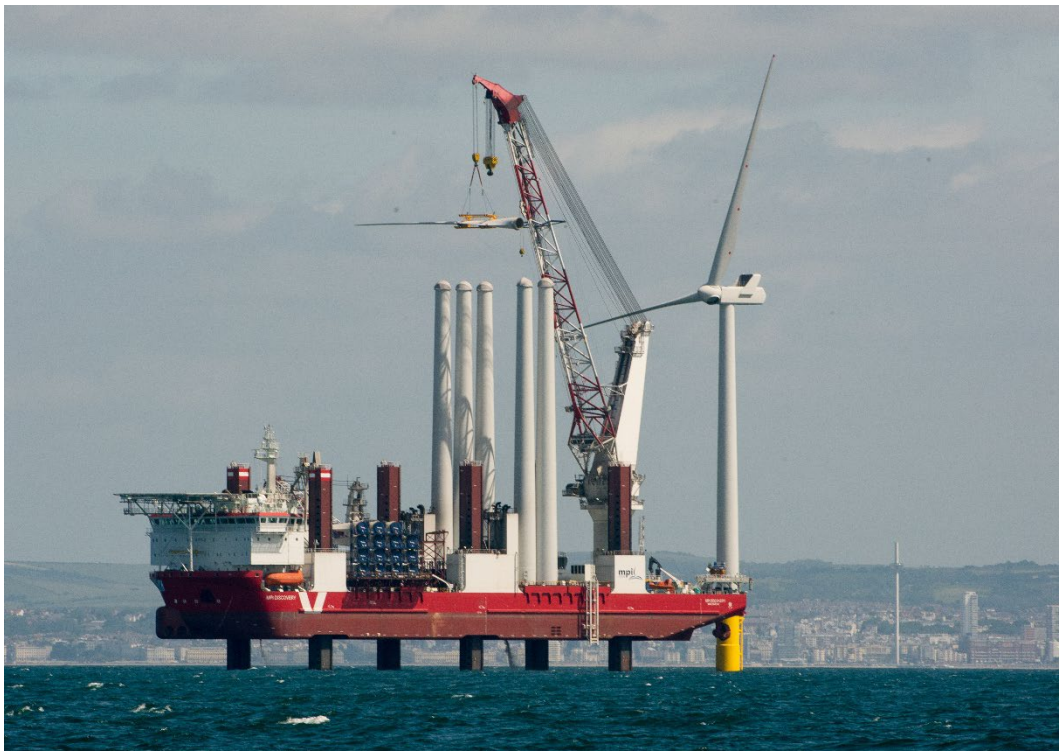
Graphic 4-4 Example jack-up vessel installing a wind turbine (Rampion 1 offshore wind farm)
